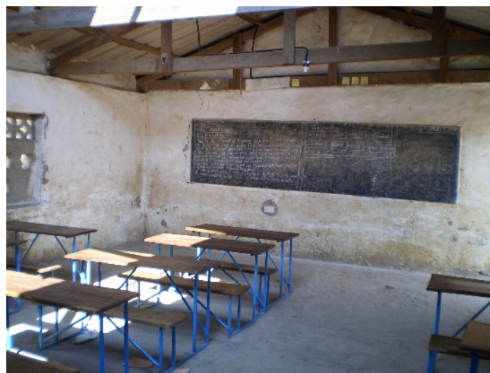
A typical classroom.
